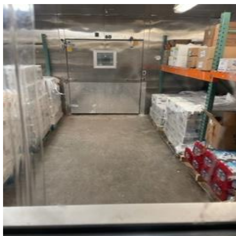
Photo: 29 Cold Storage
