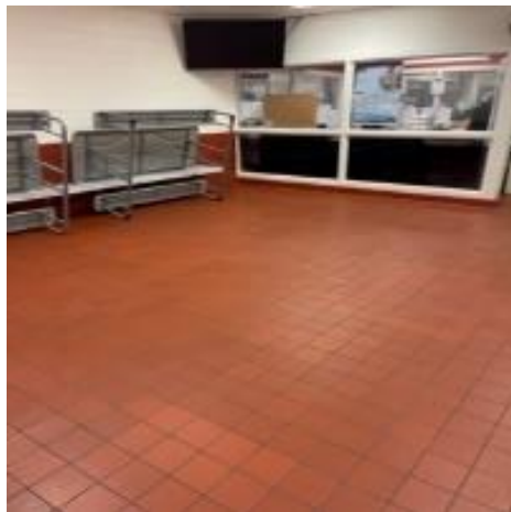
Photo: 27 Kitchen Area Clean Floor
